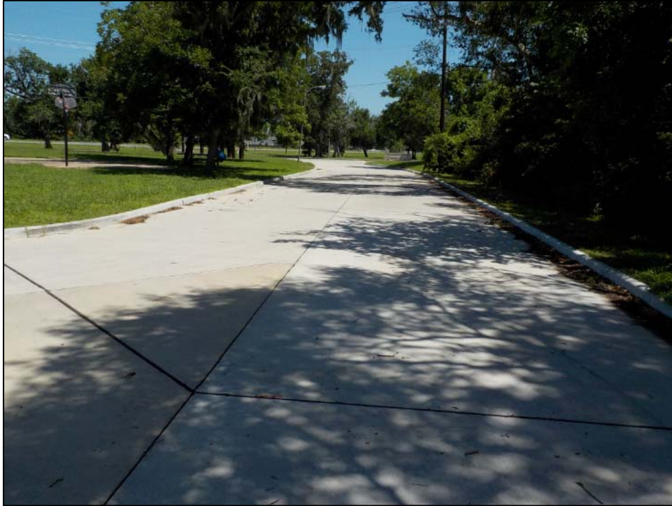
Photo 3. View along Briarcrest St within the subdivision, facing north.
