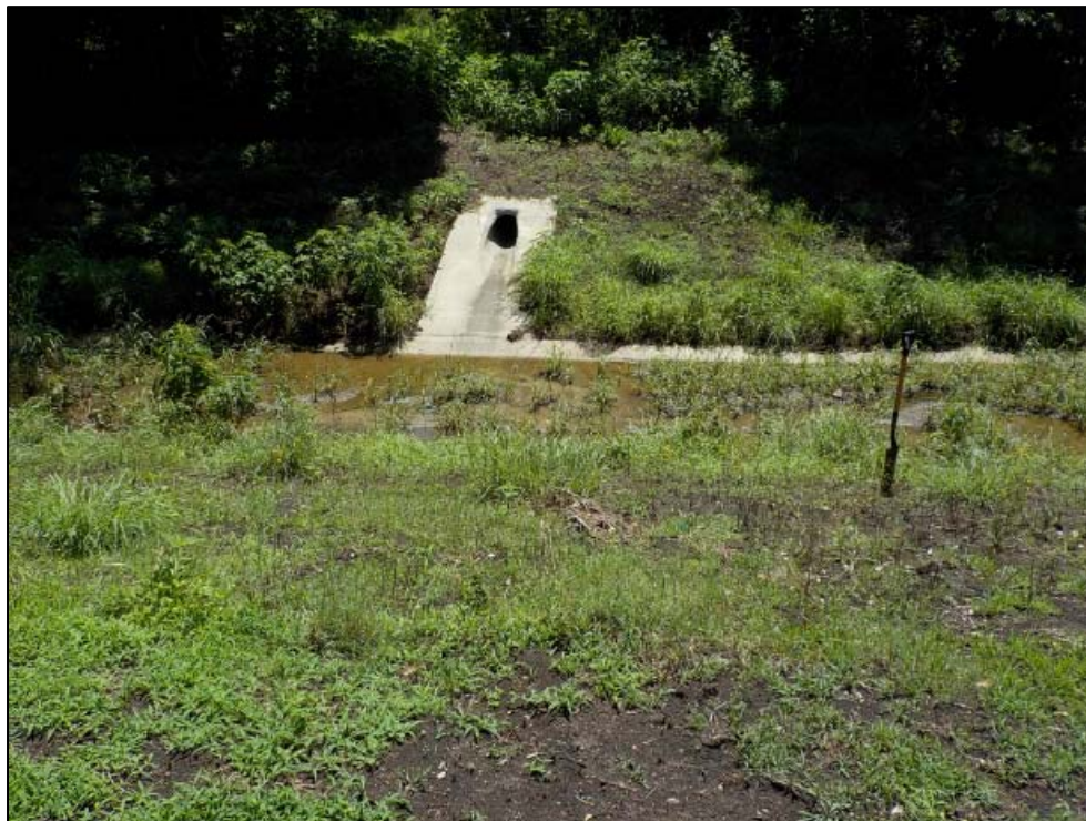
Photo 10. View across the Ditch 1 channel near the north end, facing east.
