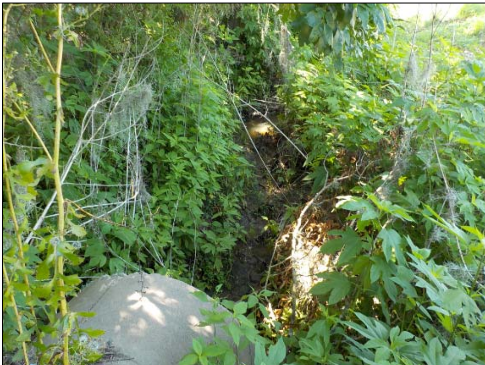
Photo 16. View of the upstream end of Ditch 2 (stormwater drainage ditch), which originates from a stormwater outfall pipe from the subdivision storm sewer system, facing south (downstream).
