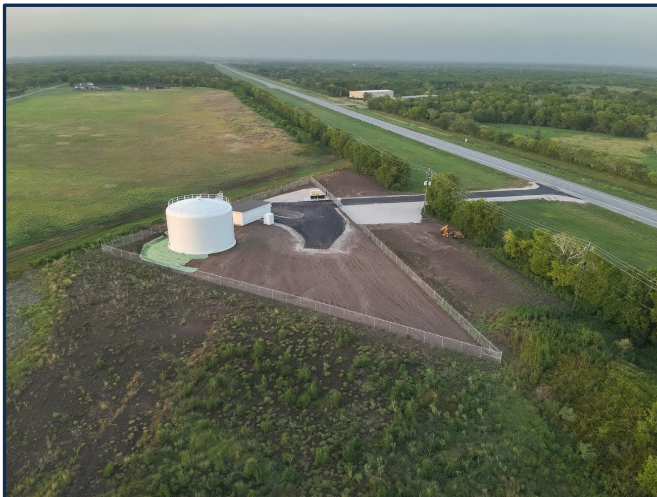
North Water Plant, a $4 million project, will see completion and come online in FY24.
